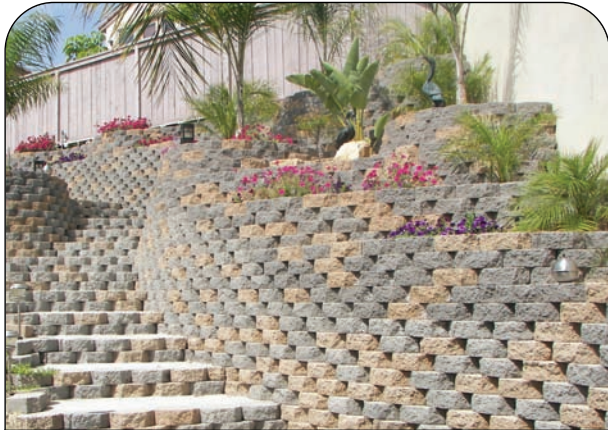
Retaining or Terrace Walls
